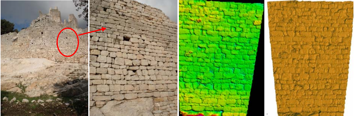
Figure 4: S.Silvestro rock near Piombino (Italy) and the detailed 3D modeling of its rock walls, simply from 3 convergent images acquired with a consumer grade digital camera with 6 Mega pixels.
